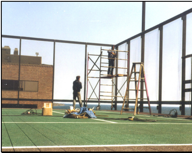
Rooftop maintenance project in the Midwest
